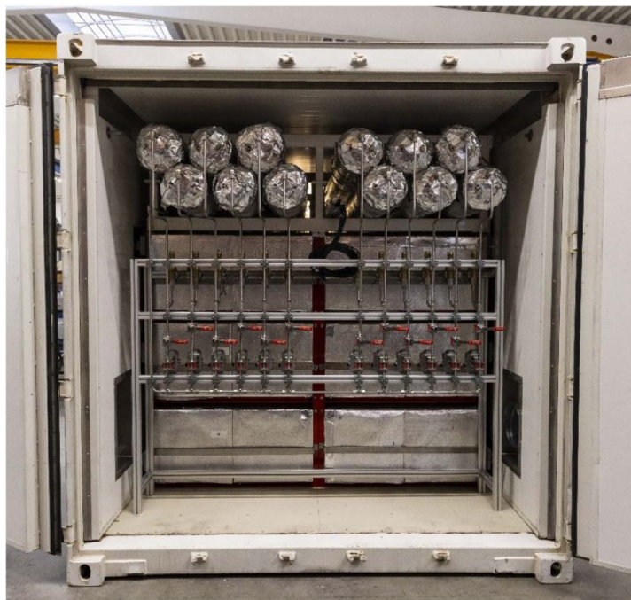
Figure 23. HyCARE system: cylinders at the top contain the metal hydride for hydrogen storage and boxes at the bottom contain the PCM for heat storage.
